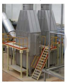
A cold plasma installation removing odour and particulates from industrial emissions.
